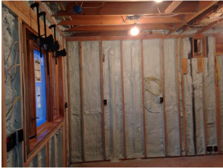
New spray foam insulation in existing walls.
