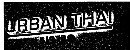
Backlighting behind individually mounted letters (Allowed)
