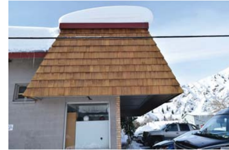
EXISTING SHAKES ROOF
