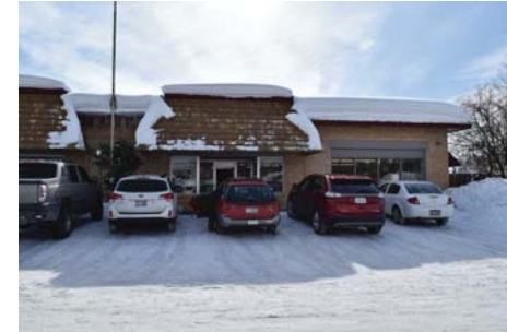
EXISTING STORE FRONT
