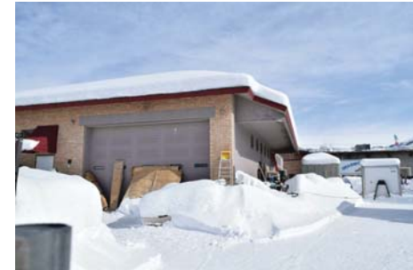
REAR OF THE BUILDING-EXISTING
