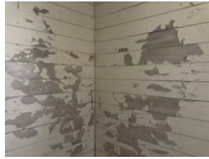
9. SALVAGE & REPURPOSE 1x6 WOOD WALL PLANKS - TYP.
