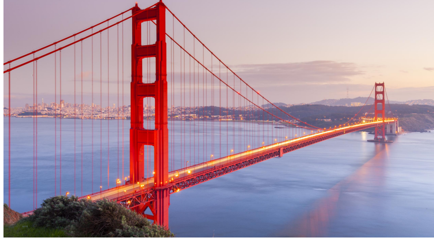
Golden Gate Bridge in San Francisco, California. Source: VisitTheUSA
