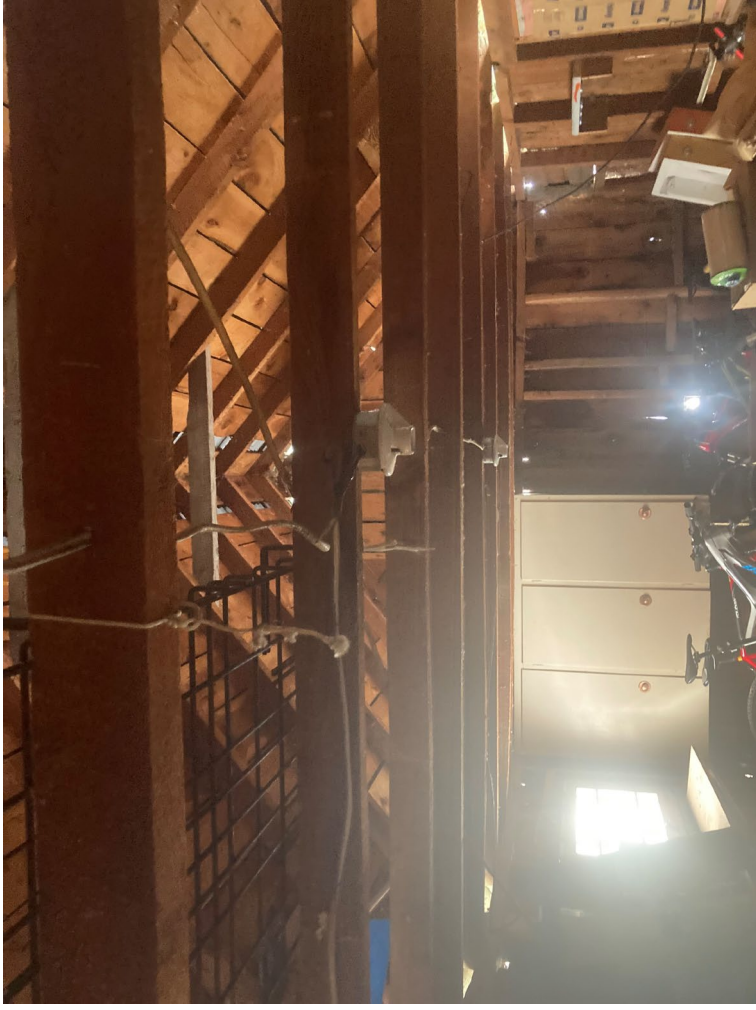
North Shed Interior – 2x4 Rafters & Collar Ties
