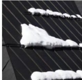
MATTE BLACK METAL ROOF WITH SNOW RETENTION
