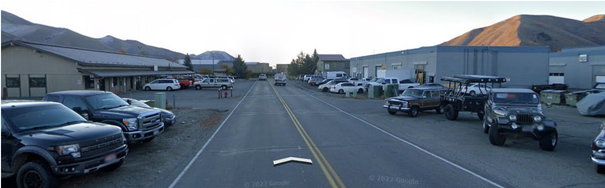
Airport Way, looking directly south from the project site.
