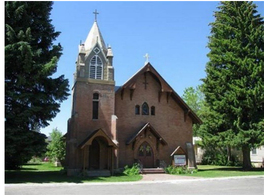
Figure 2- Existing Bell Tower, Church and Spruce Trees
