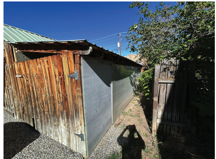
SOUTH VIEW OF EXISTING GARAGE
