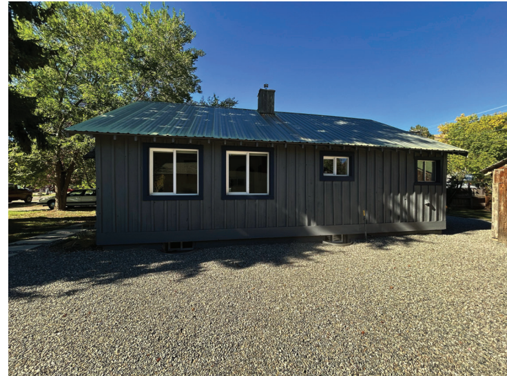
SOUTH VIEW OF EXISTING HOUSE- TO BE RETAINED
