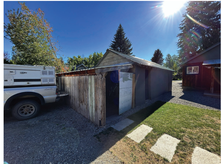
ALLEY VIEW OF EXISTING GARAGE
