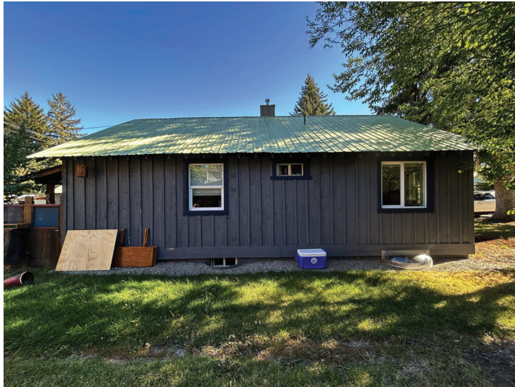
NORTH VIEW OF EXISTING HOUSE- TO BE RETAINED
