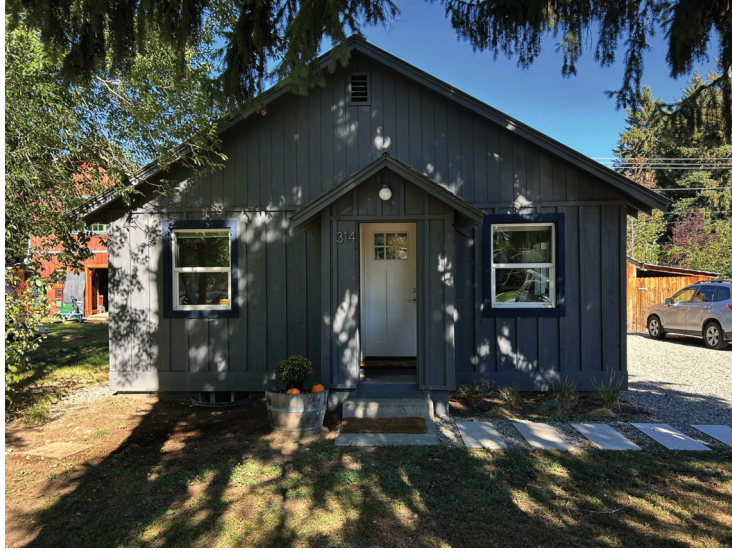
FRONT VIEW OF EXISTING HOUSE- TO BE RETAINED
