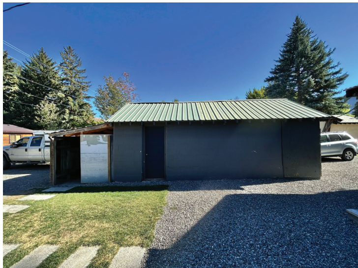
NORTH VIEW OF EXISTING GARAGE
