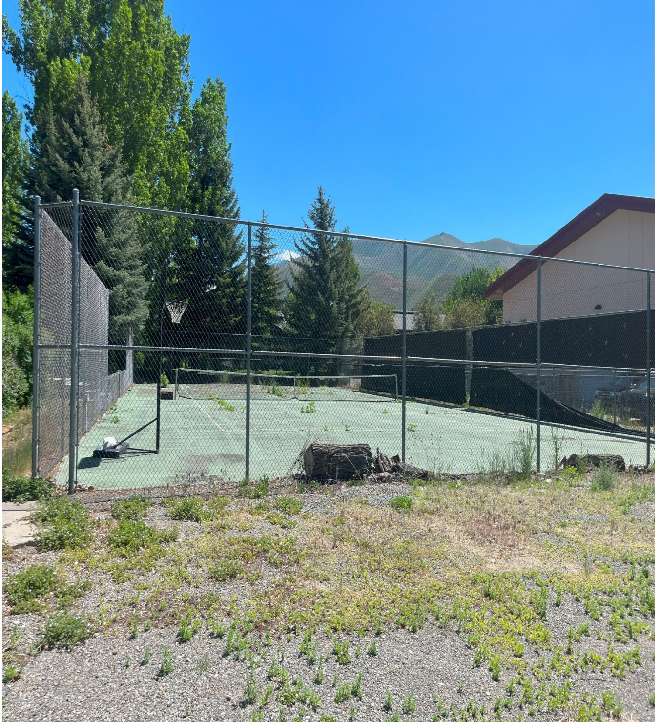
FIGURE 3. EXISTING TENNIS COURT TO BE DEMOLISHED
