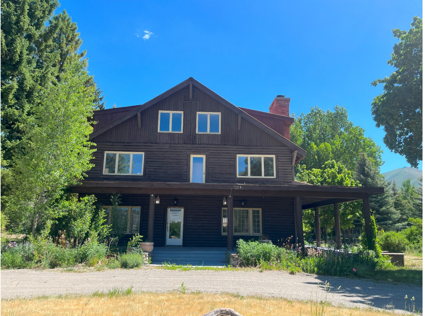
FIGURE 1. EXISTING INN TO BE RENOVATED
