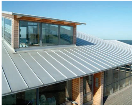
STANDING SEAM METAL ROOFING
