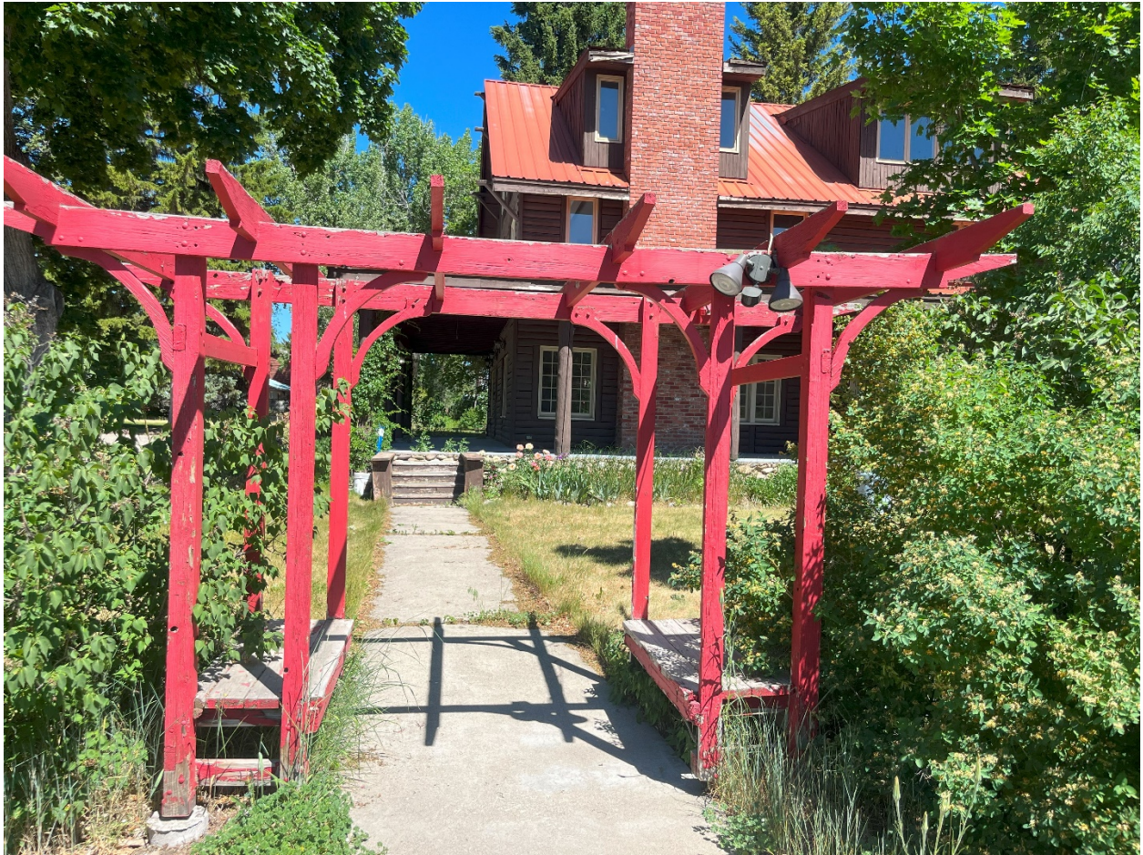
FIGURE 4. EXISTING STRUCTURE TO BE DEMOLISHED
