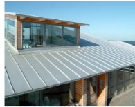
STANDING SEAM METAL ROOFING COLOR: ZINC GRAY
