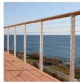
METAL CABLE BALUNING WITH WOOD LAG
