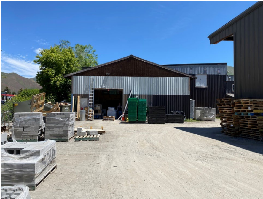
WEST ELEVATION (PARTIAL) – ADDITION TO STORAGE WILL BE TO SOUTH (RIGHT)
