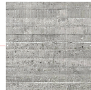
CAST IN PLACE BOARD FORM CONCRETE WALL
