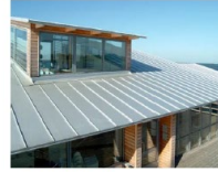
STANDING SEAM METAL ROOFING COLOR: ZINC GRAY
