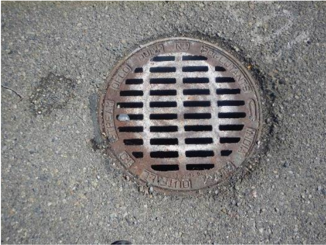
Photo 5: Close up of storm drain
