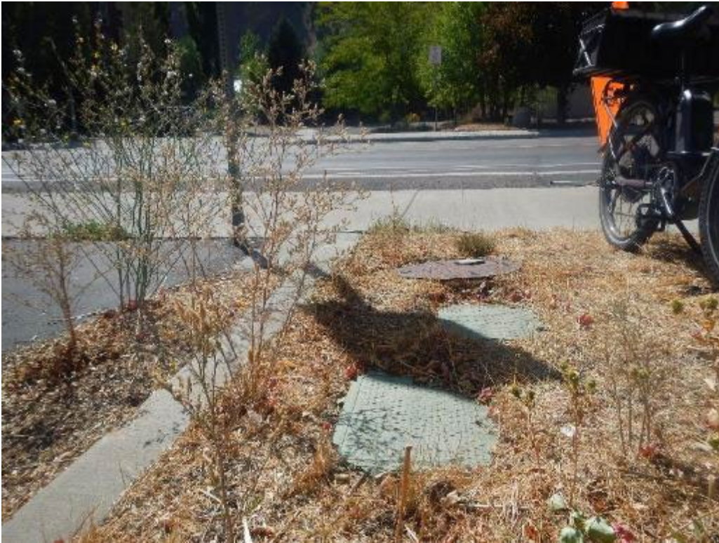
Photo 17: water meter and irrigation control boxes on old cinema parking lot across River Street Note: Mr. Williams advised that city water extends to the subject property under River Street from this meter
