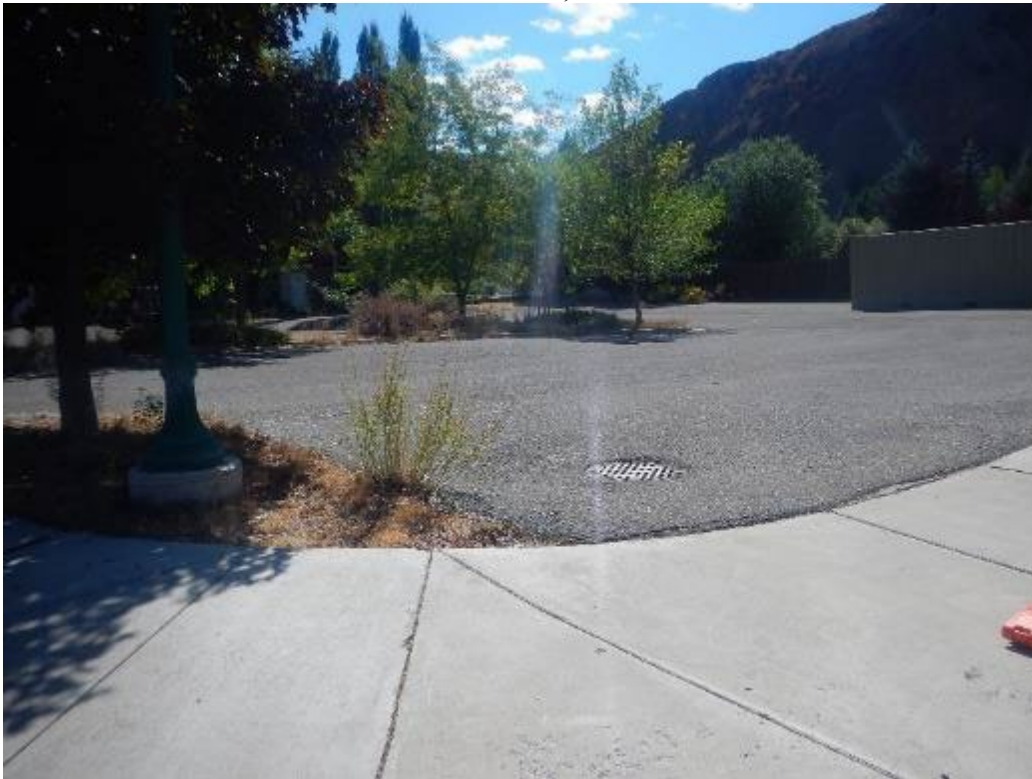
Photo 4: Looking SW across subject property Note: one of two storm drains on subject property; this one appears to be in higher area so would not likely receive much drainage.
