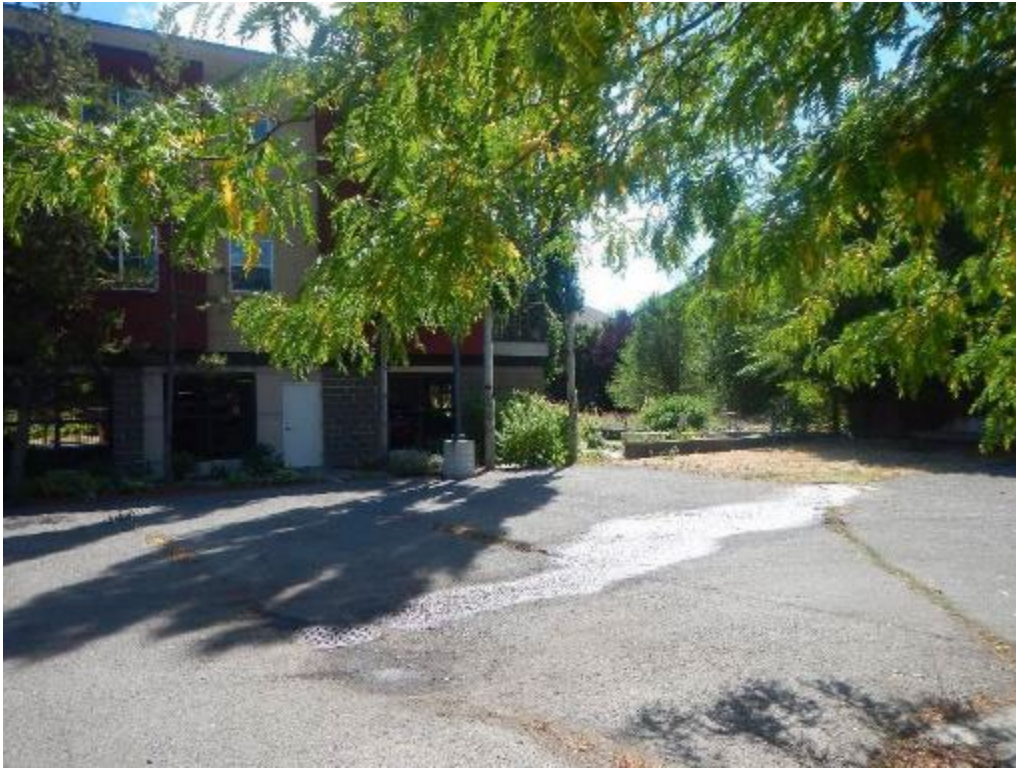
Photo 7: 2 nd storm drain observed on subject property
