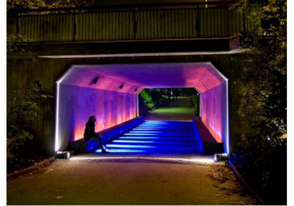
Lit Pedestrian Tunnel at Night
