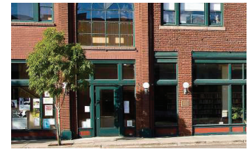
⑦ EXISTING ENTRY OFF MAIN ST TO CITY HALL
