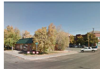
⑤ EXISTING CITY BUILDING (TOWN CENTER WEST)
