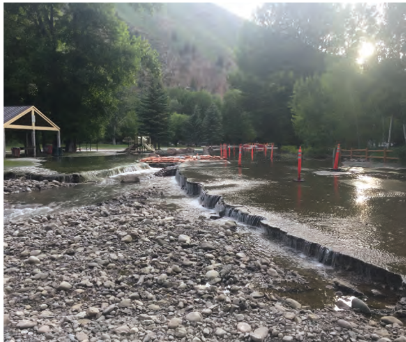
2017 FLOODWATERS BEING CONVEYED DOWN WAR EAGLE AND AROUND HEAGLE PARK
