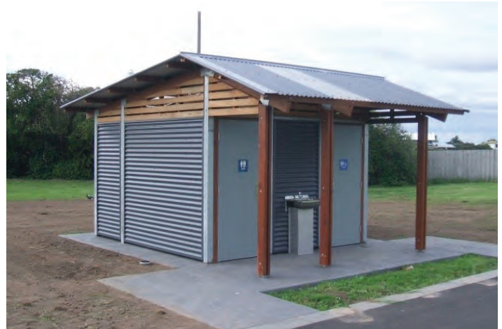
TYPICAL PUBLIC RESTROOM AT A CITY PARK
