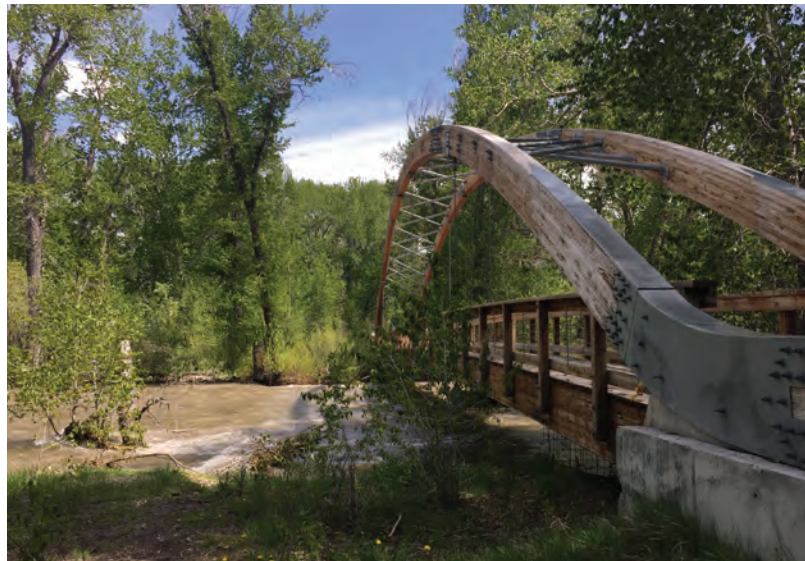
EXISTING PEDESTRIAN BRIDGE WITHIN THE GREENWAY
