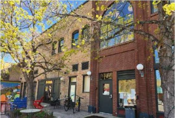
2 EXISTING STAIR/SECONDARY REAR ENTRY TO CITY HALL & CHILDREN'S LIBRARY
