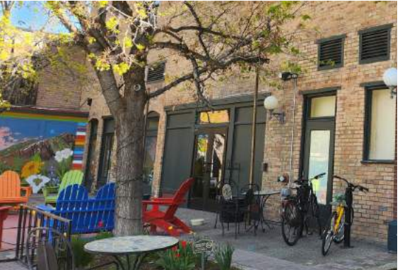
8 EXISTING REAR ENTRY TO CHILDREN'S LIBRARY
