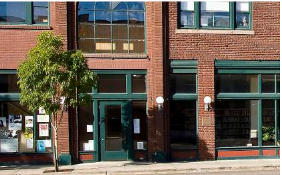
7 EXISTING ENTRY OFF MAIN ST TO CITY HALL
