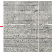
CAST IN PLACE BOARD FORM CONCRETE WALL
