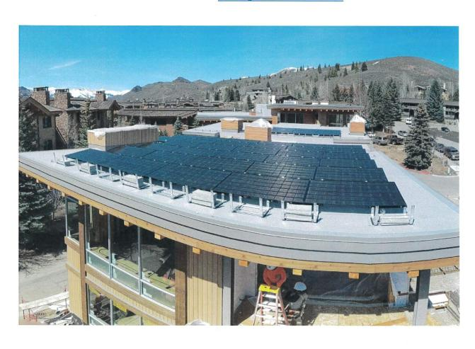
The following is a proposal for a grid-tied solar array at Hailey City Hall. This proposal is for 85 x Canadian Solar 400 watt (or equivalent) solar panels. For 85 panels, the system would be sized at 34 kW of solar. This system is priced at \$3.19/watt.
