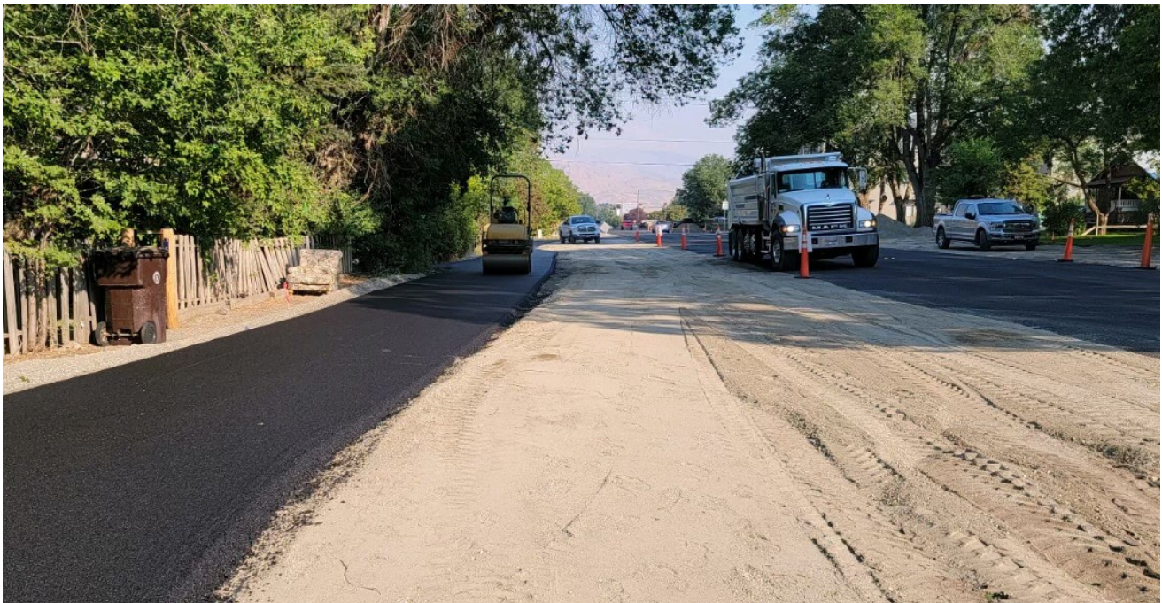
RIVER STREET PATHWAY INSTALL PROCESS
