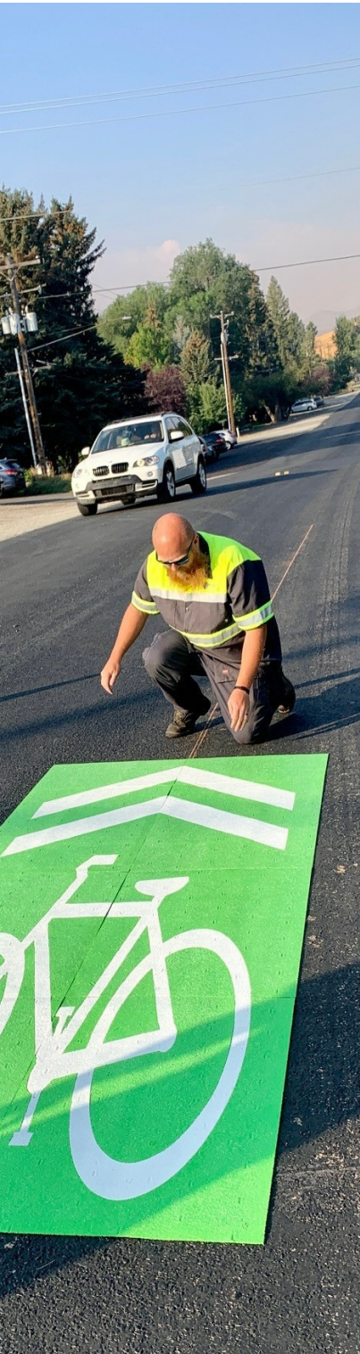
"SHARROW" INSTALLATION ON W BULLION ST
