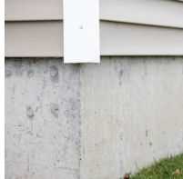
Foundation Exposed (grey) Concrete
