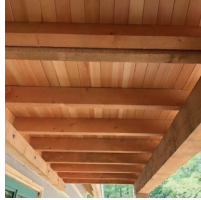
Exposed Canopy Roof Soffits 1/2" X 3-1/2" cedar T&G tight knot pre-stained
