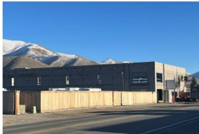
New Construction at approximately 1120 Airport Way (Aviation Drive)
