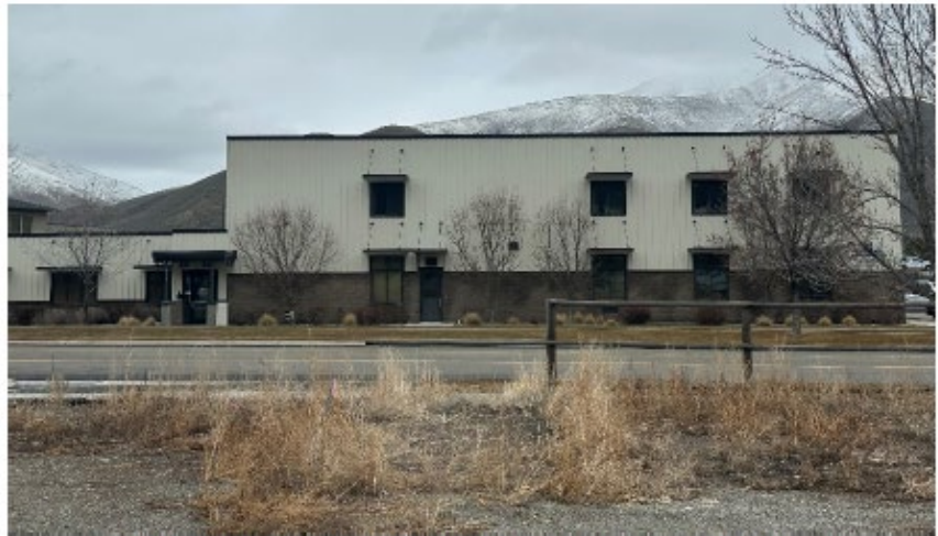
1630 Aviation Drive (Existing Building Immediately across the street)
