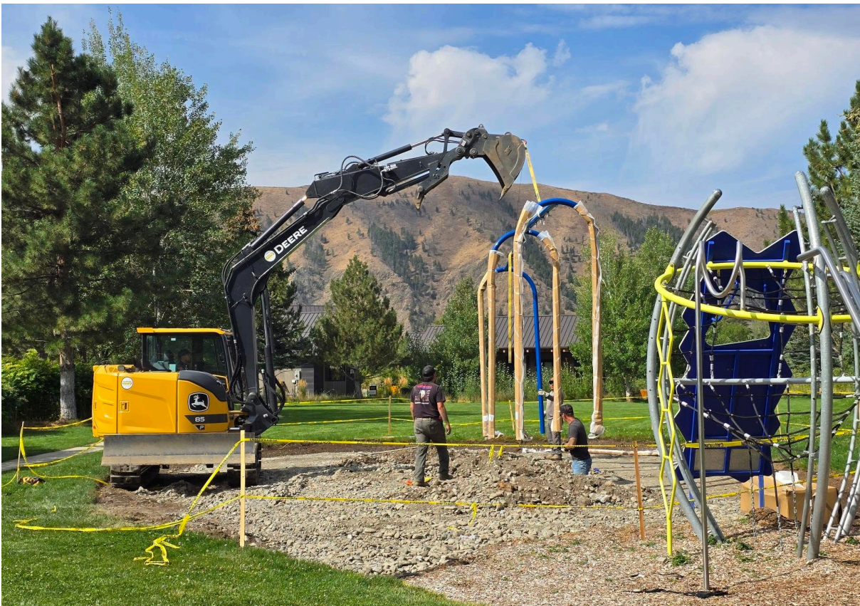
NEW SWINGSET BEING INSTALLED AT OLD CUTTERS PARK
